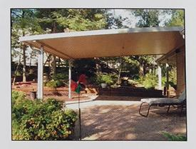
These covers are constructed with a 3 inch panel made up of styrofoam insulation with aluminum on both sides. This style is perfect for a patio that may be eventually enclosed. Available in white or ivory.
